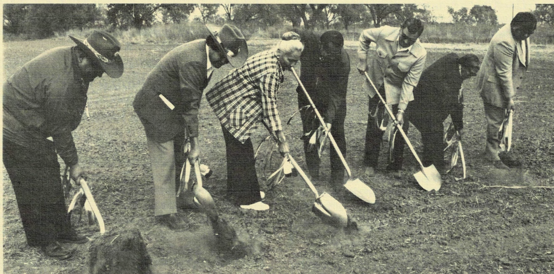
AFTER MORE THAN ten years of planning and preparation, construction of the new Anadarko Indian Health Clinic in Anadarko, Okla., officially commenced with ground-breaking ceremonies October 25. Pictured (l-r) here are representatives from the seven Oklahoma tribes that will be served by the clinic: Neil Wooster, Caddo Tribe; Edgar French, Chairman, Delaware Tribe; Mildred Cleghorn, Chairman, Ft. Sell Apache Tribe; Lonnie Tsoataddle, Chairman, Apache Tribe; Glenn Hamilton, Kiowa Tribe; George Watchetaker, Comanche Tribe; and Newton Lamar, Chairman, Wichita Tribe. NIH Oklahoma City Representative Lawrence Snake presided over the ceremonies. (Photo Courtesy Jim Cussen, IHS Liaison Officer)
